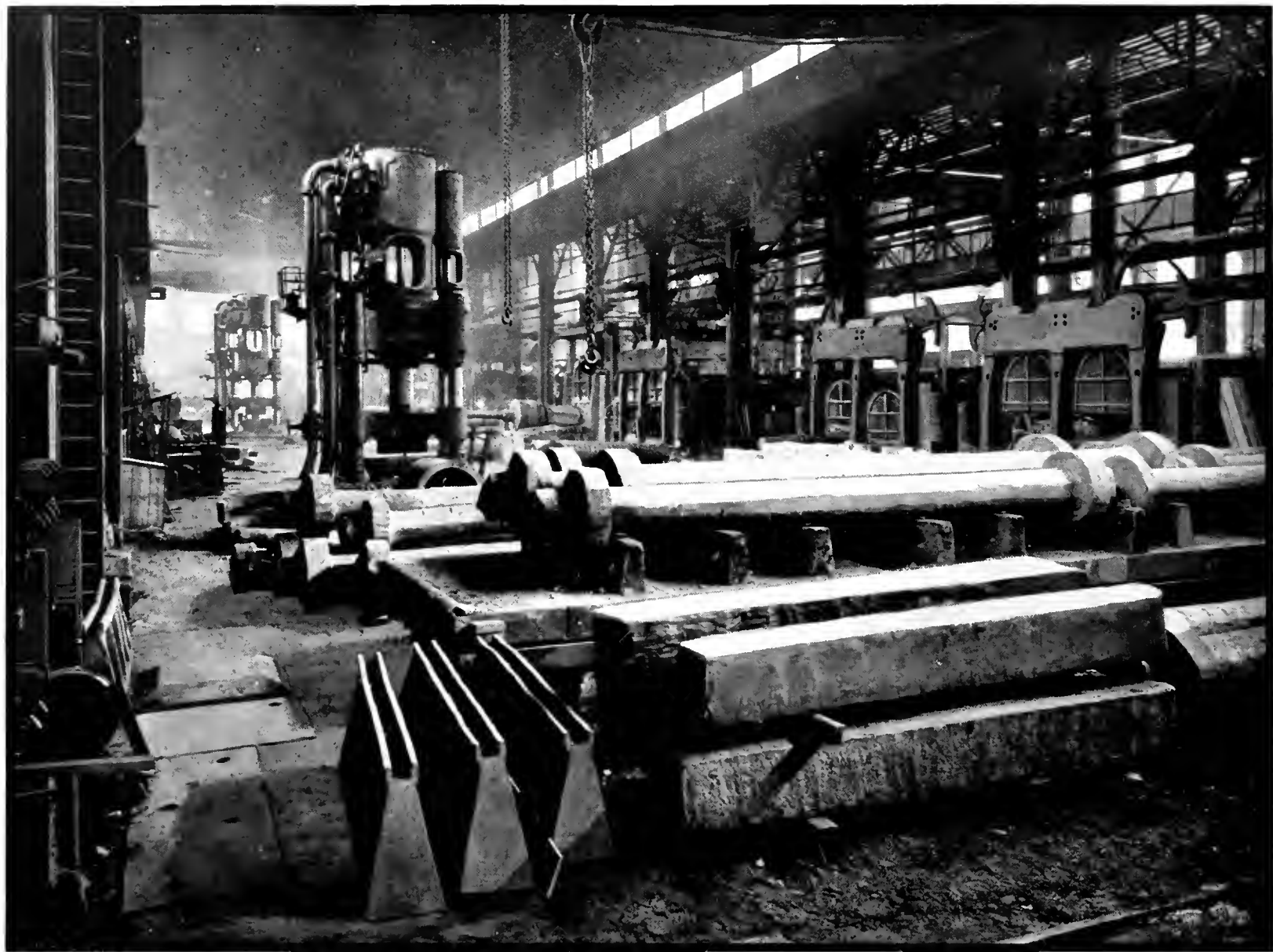
Forge Department No. 2, Showing Two 1500-Ton Steam Hydraulic Forging Presses
